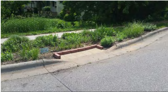
Figure 5 New inlets to replace difficult to maintain rock inlets installed by the City.
