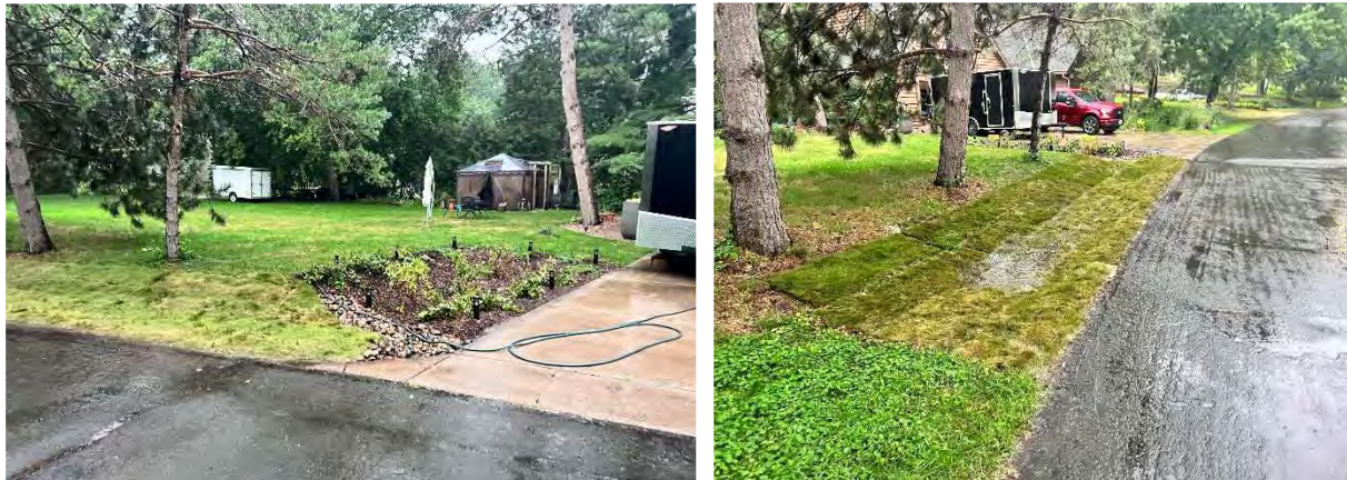
[Above] Riviera Avenue Treatment Train Bioretention.
