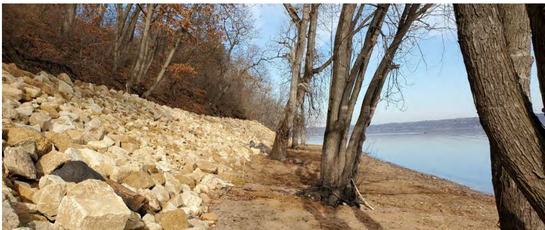
[Above] Lake St. Croix Beach bluff toe stabilization.
