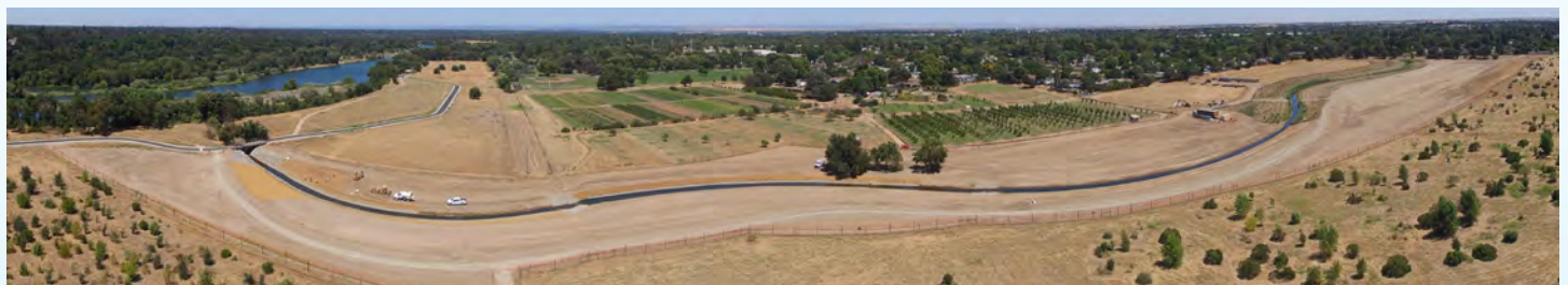
Cordova Creek - Phase II designs are currently in progress to restore the last section of channel (left) to provide fish passage to the lower American River
