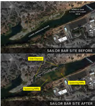
Lower American River – Upper Sailor Bar site before and after side channel installation.
