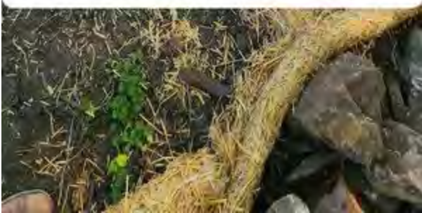
Oats and blanket applied, double reinforced silt fence in place
