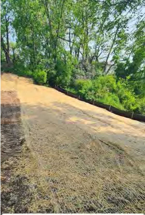
Oats and blanket applied, double reinforced silt fence in place
