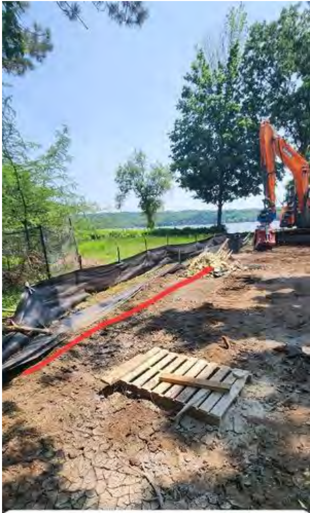
Repair redundant silt fence here
